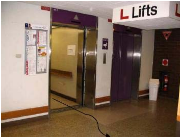
Figure 7: There is a 30° 'S' turn after exiting the lifts on Level 2 which enters into a corridor.
